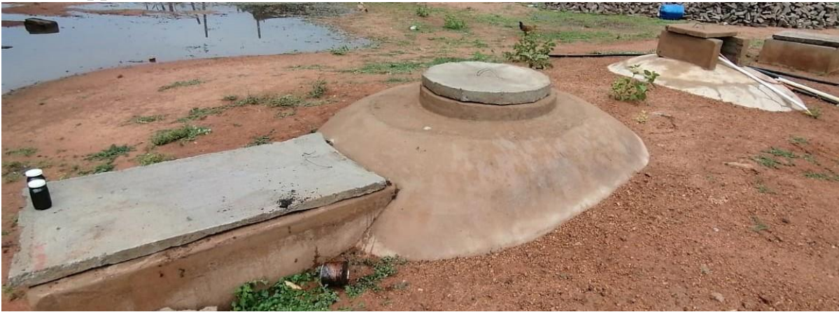
Figure 1a: Biogas plant at Nnone farm, Ramaphatle
